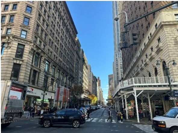
Photo 4-3 Eastward View of West 34th Street from Sixth Avenue
