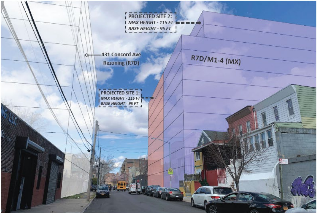
2 Looking northeast along Concord Avenue toward the Rezoning Area
