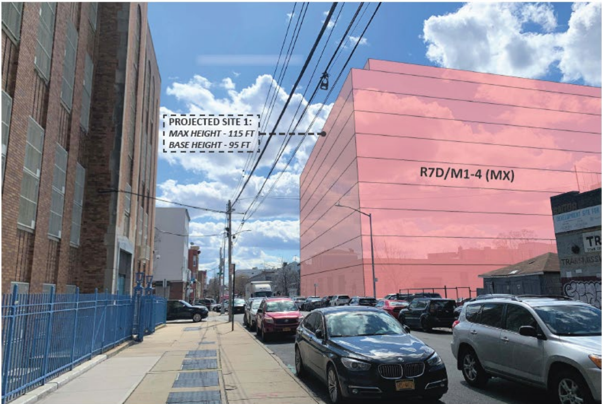
3 Looking south toward the intersection of E 145 Street and Wales Avenue
