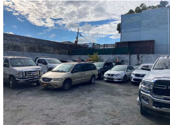
20 Minor staining seen in the pavement at 438 Concord Avenue.
