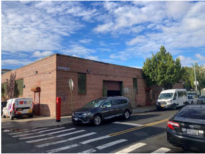
01 View of 435 Wales Avenue facing southwest.
