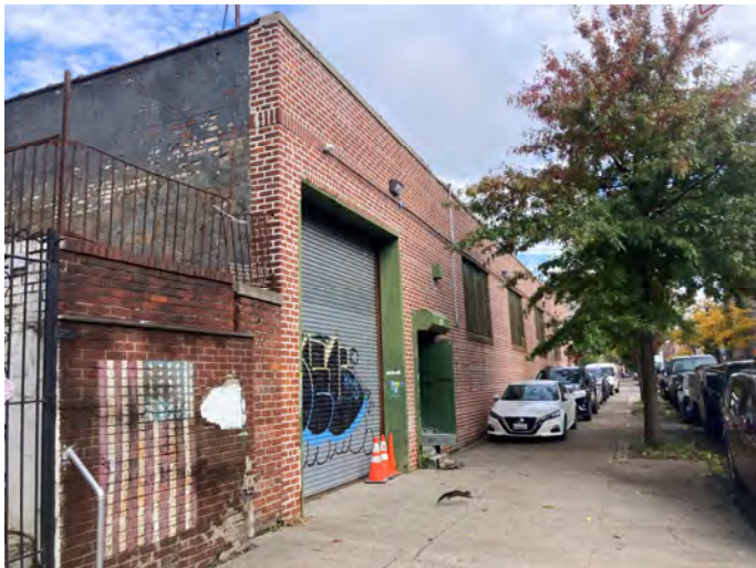
03 View of a garage door at 435 Wales Ave facing north.
