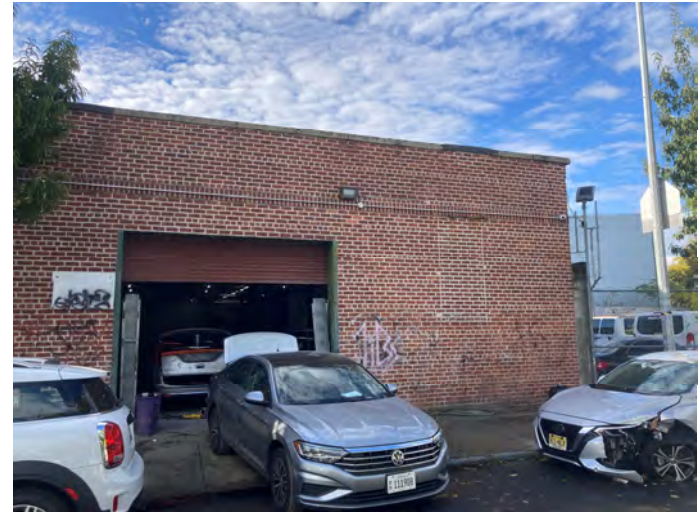
02 View of a garage door at 435 Wales Ave facing south.
