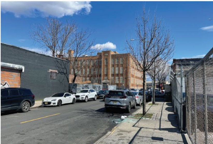
5 View of Mott Haven Community High School from East 145 St facing east
