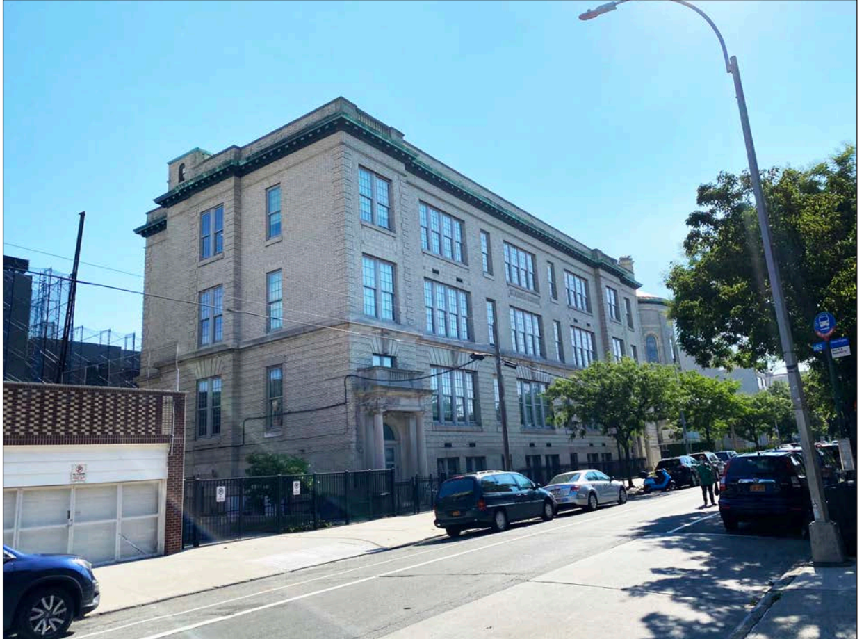
The former St. Joseph's School, at 638 Dean Street 11
