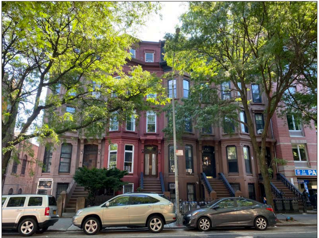
View southeast on Washington Avenue to residential buildings in the Clinton Hill South Historic District 6
