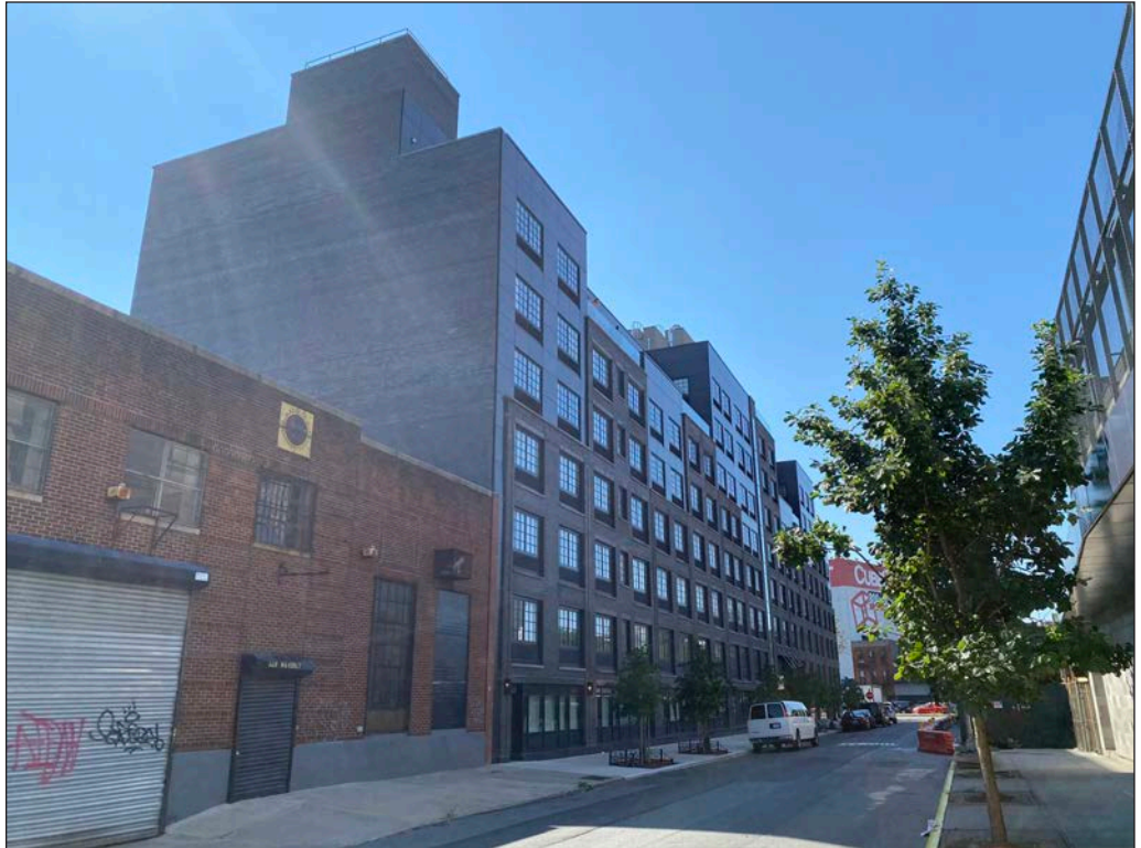
View southeast along Waverly Street, from north of Atlantic Avenue 5
