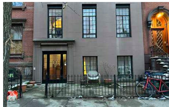
EXISTING ENTRANCE AREA - PHOTOGRAPH
