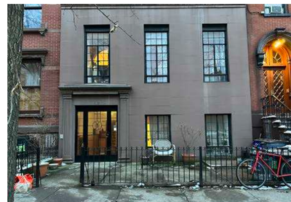
EXISTING ENTRANCE AREA - PHOTOGRAPH
