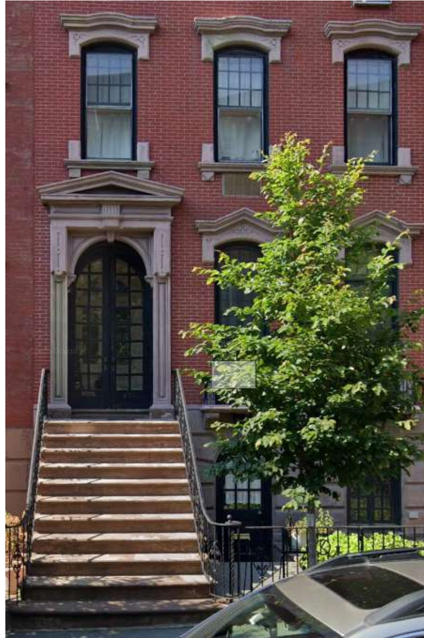
STOOP #2: 139 NOBLE STREET Recommended precedent by LPC staff
