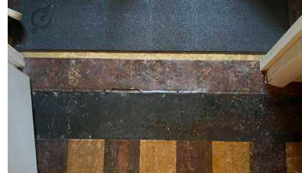
EXISTING VESTIBULE - FLOOR AND CEILING
