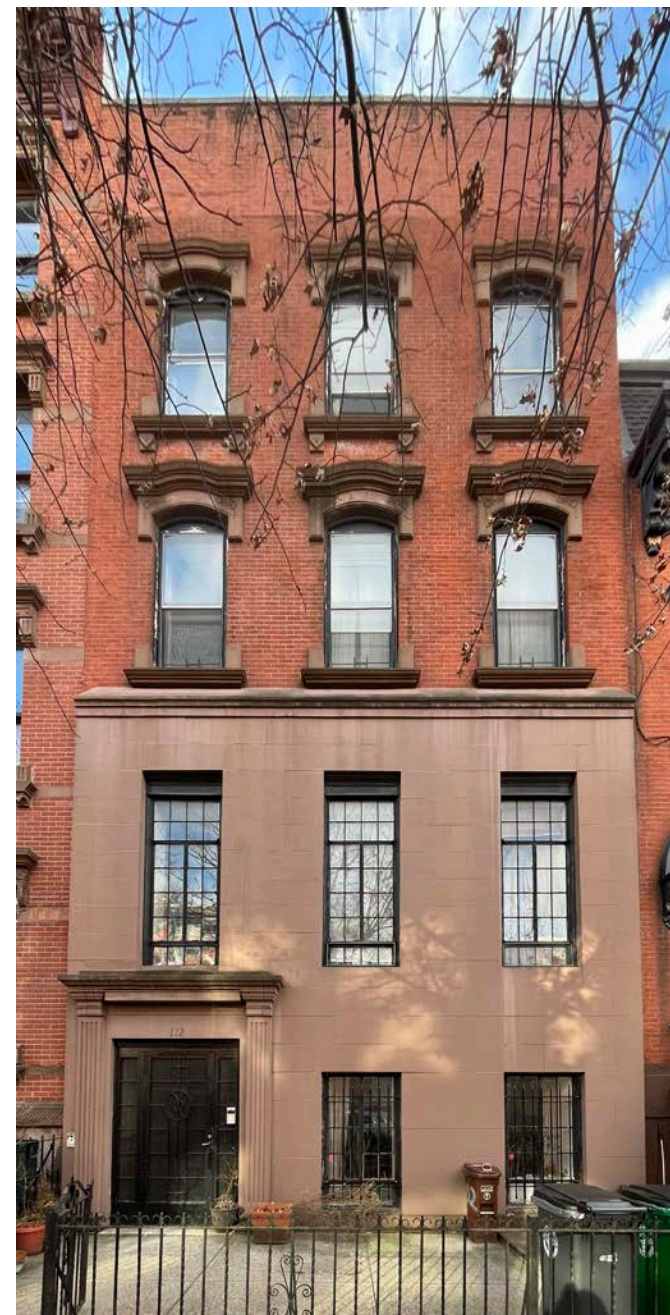
102 Kent st | Front Facade | 2025 Photo by: thread collective
