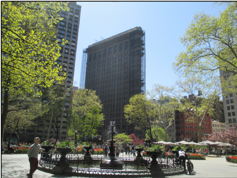
5. View of the Project Area looking southwest from Madison Square Park.
