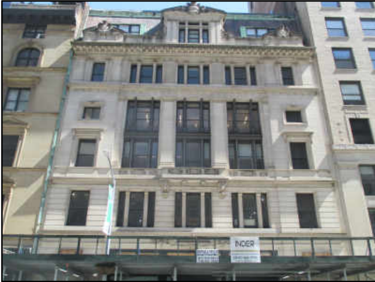
6. View of the Scribner Building looking southeast from the west side of Fifth Avenue.
