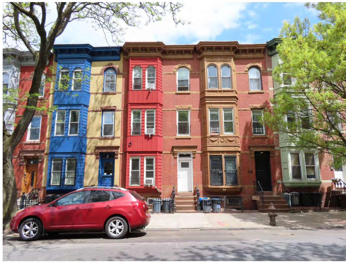
13. View of the Project Area facing northeast from Prospect Avenue.
