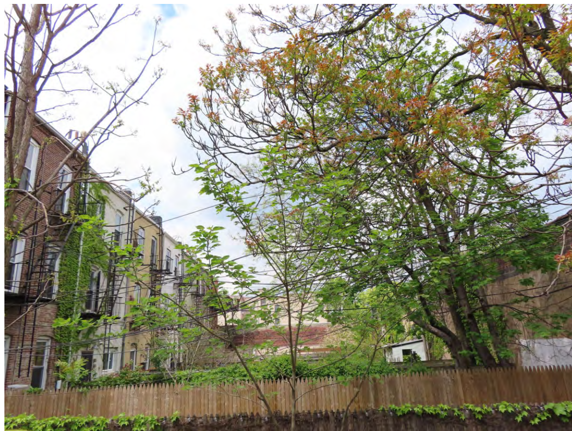
42. View of the rear of the row houses in the Project Area facing northwest from within the Development Site.
