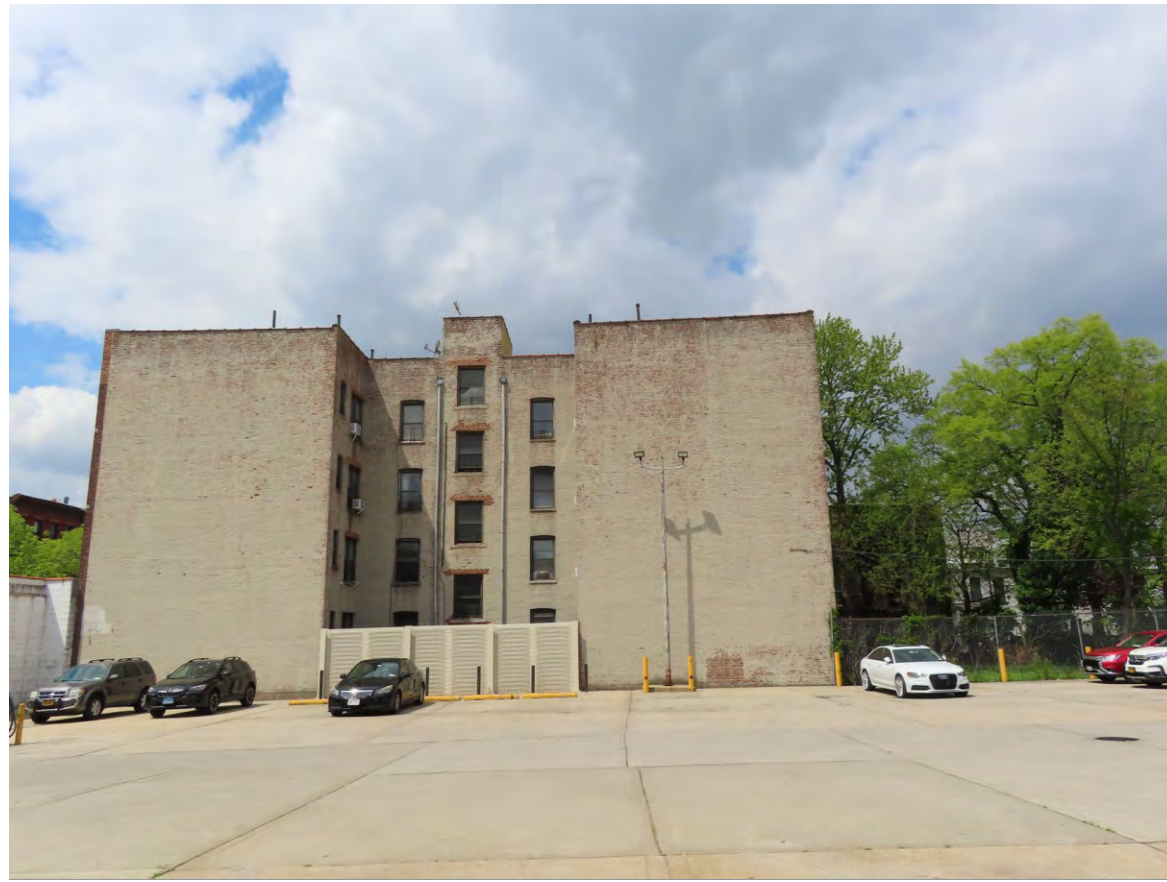
34. View from within the Development Site facing northwest.
