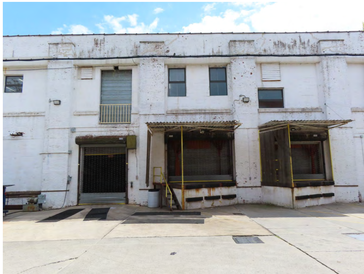
39. View from within the Development Site facing southeast.
