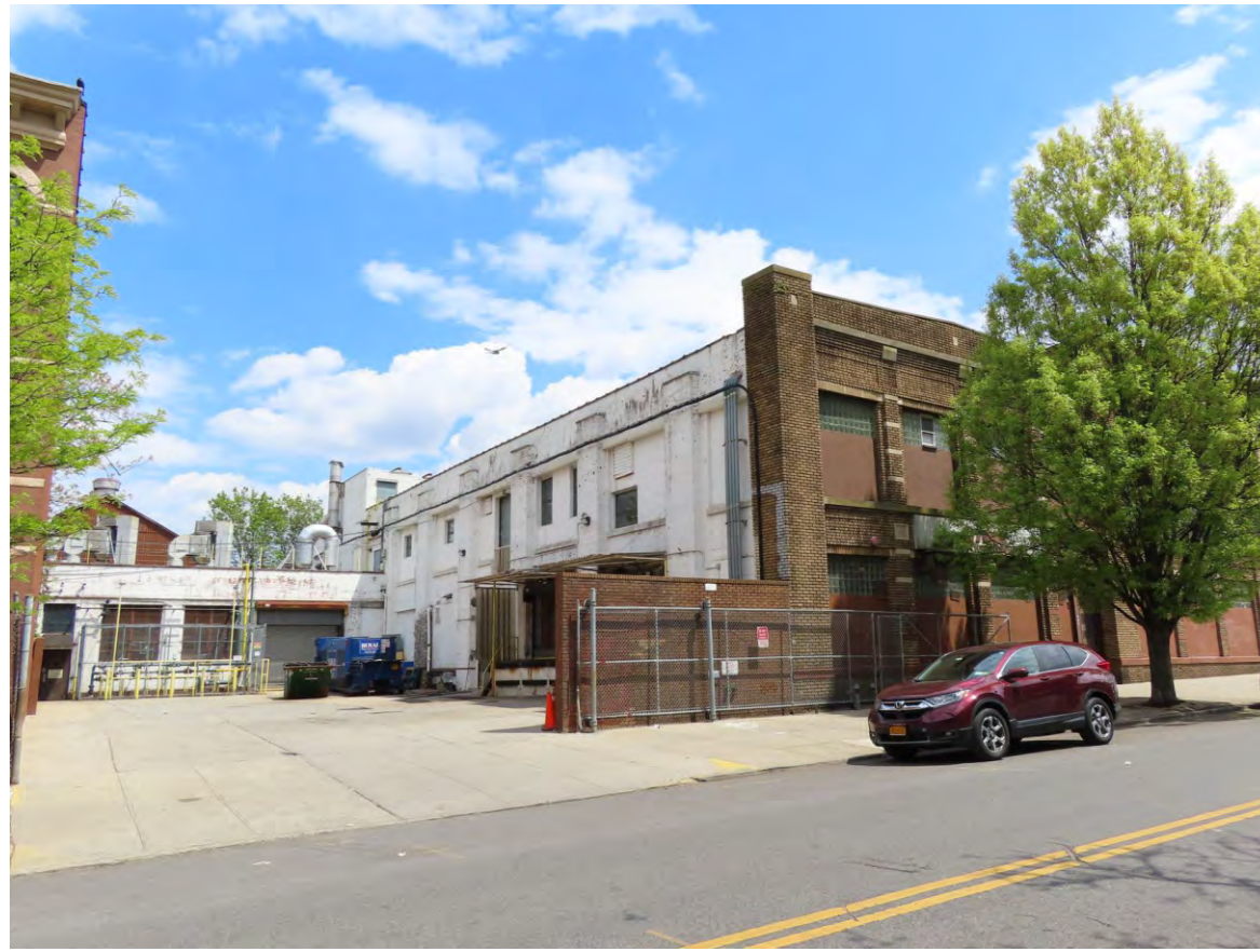
1. View of the Development Site facing east from Prospect Avenue.
