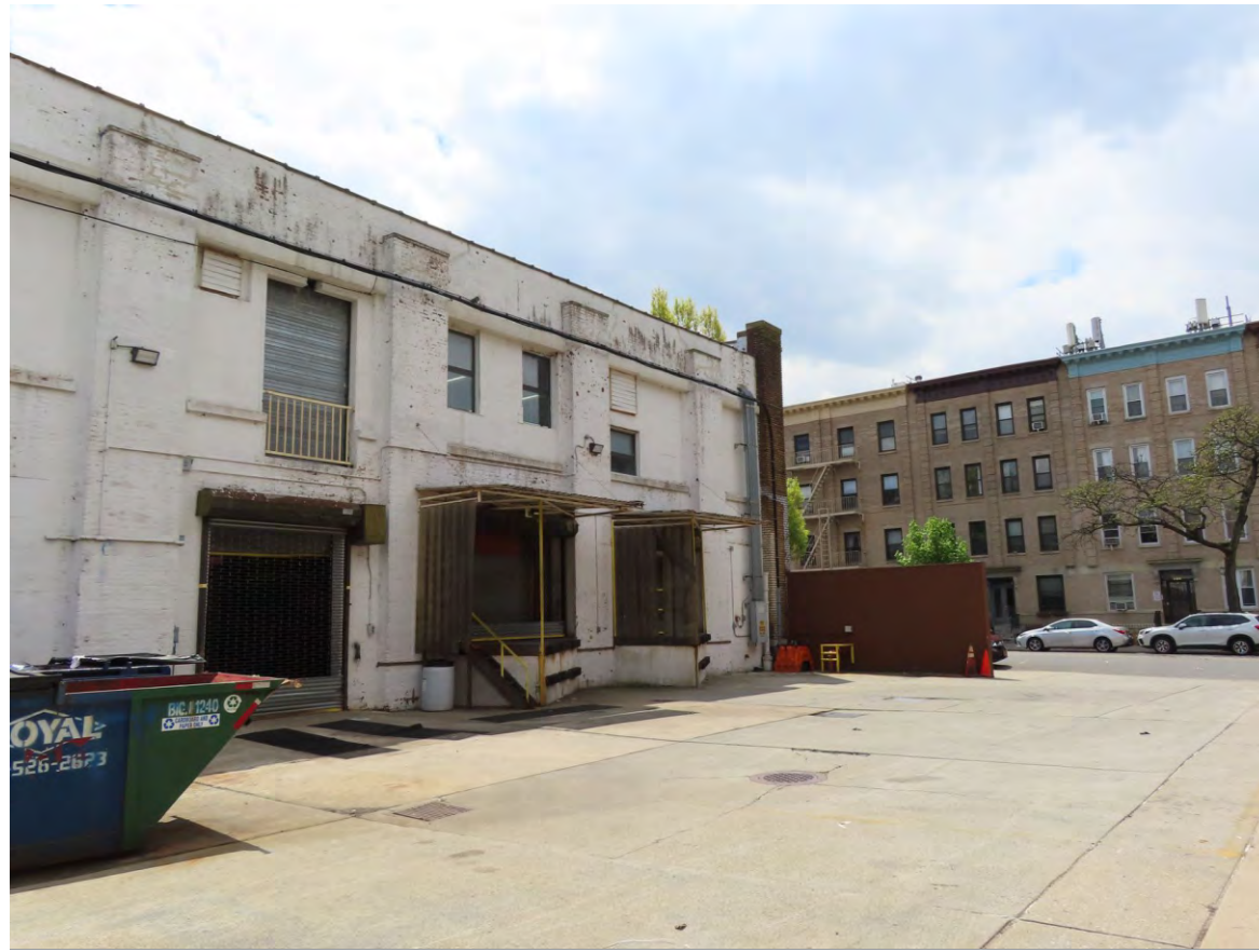
40. View from within the Development Site facing south.
