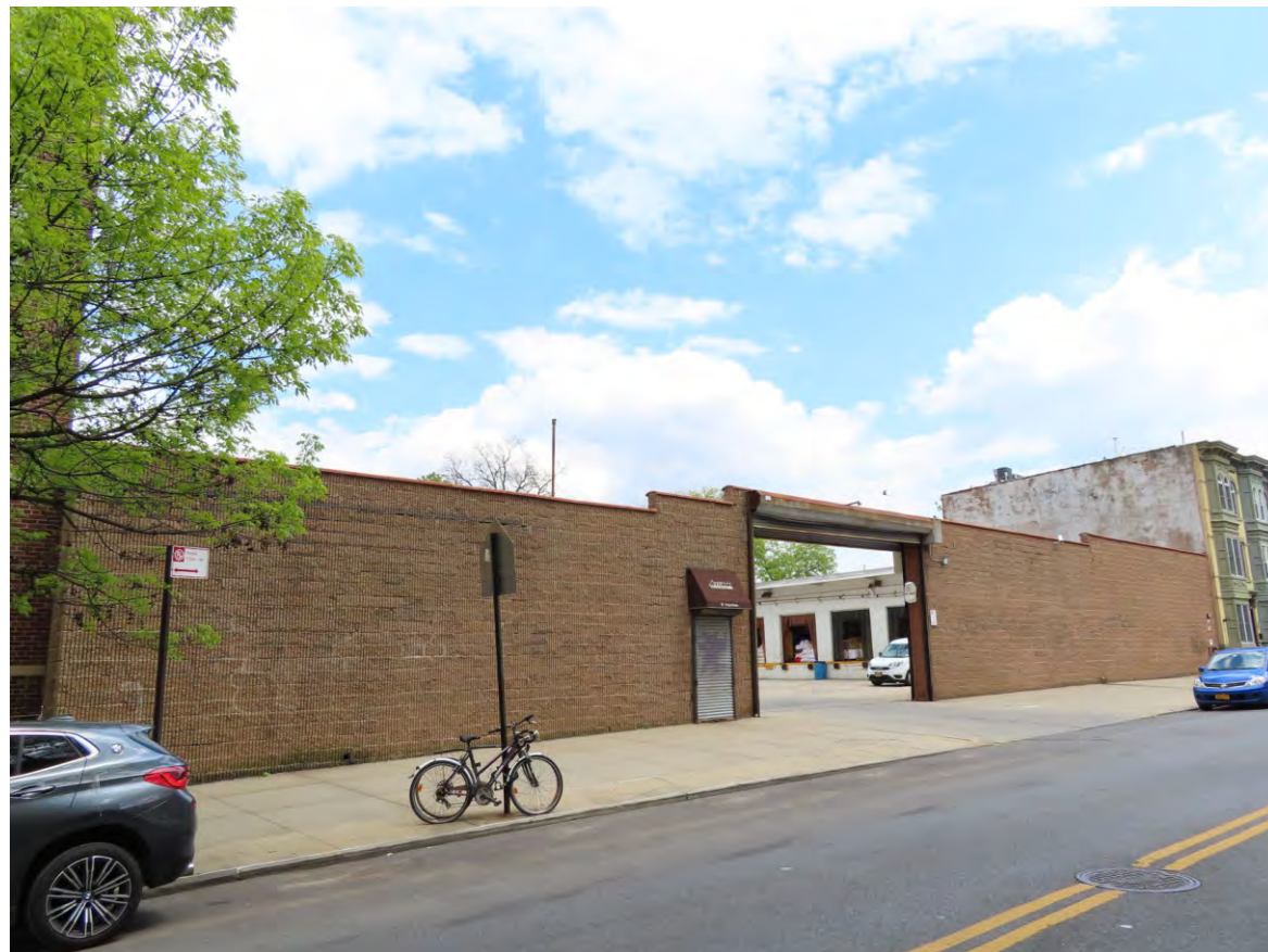
21. View of the Development Site facing east from Prospect Avenue.
