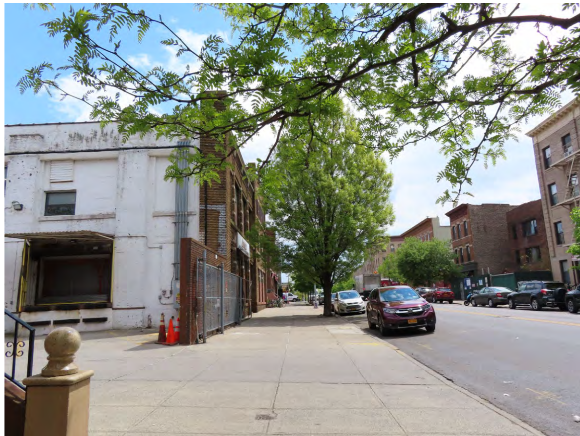
9. View of the sidewalk along the north side of Prospect Avenue facing southeast (Development Site at left).
