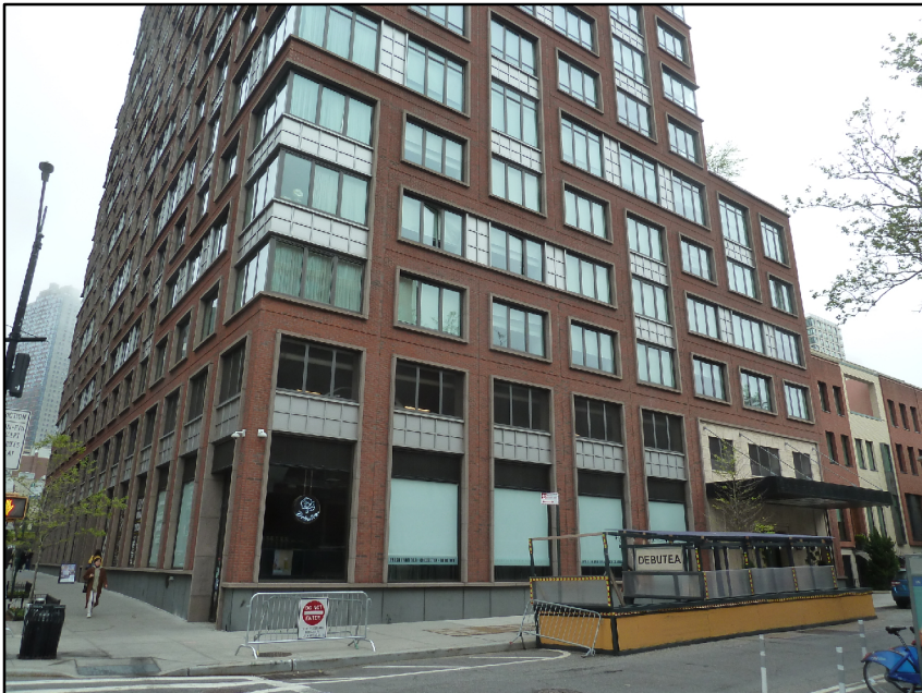
6. View looking northeast towards 140 Schermerhorn Street (Lot 7501).
