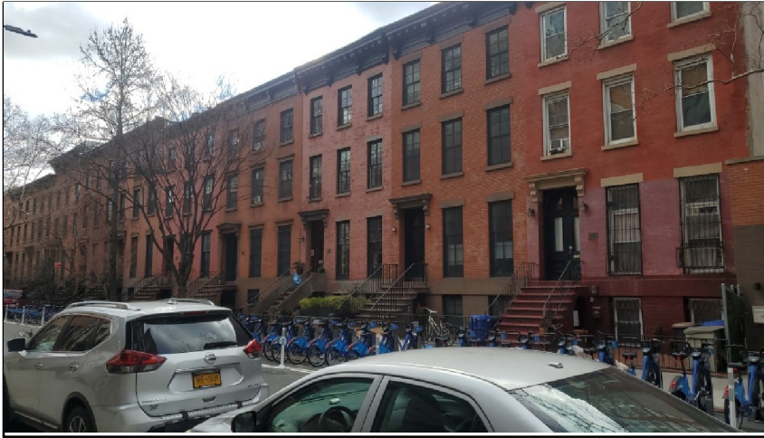
21. View looking south towards the NYCL and S/NR-listed brownstones located along State Street.
