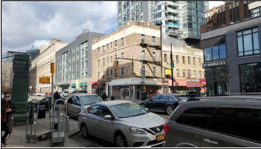
10. View looking northwest at building streetwalls near the intersection of Schermerhorn and Hoyt streets.
