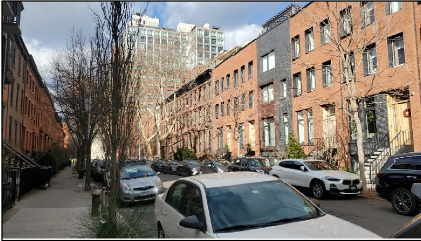
19. View looking northwest towards the NYCL and S/NR-listed brownstones located along State Street.
