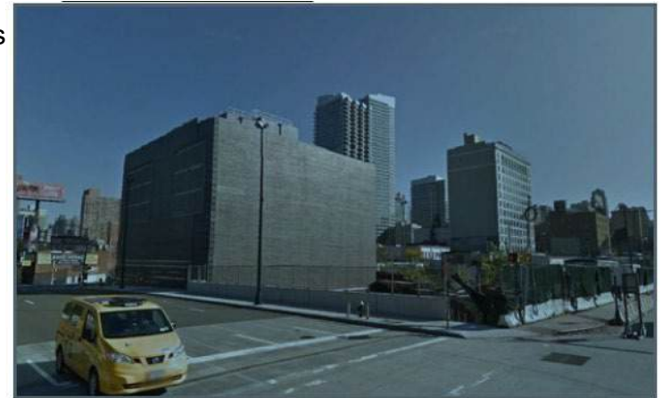
Figure 2: View of Site looking northeast from the intersection of 35 th Street and 11 th Avenue, including MTA Ventilation Shaft
